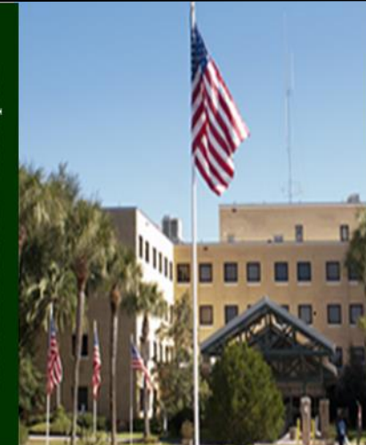
Upgrade Physical Security Malcolm Randall VA Hospital
