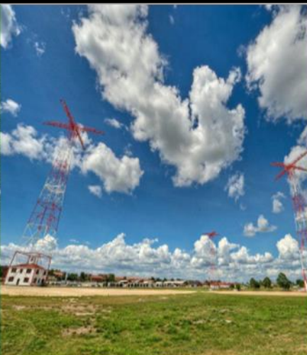
Ft. Benning Jump Towers Engineering Certification
