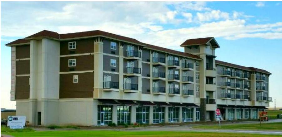
This 70,000 square foot 4-story development designed and constructed by WG Pitts Company provides retail, office, and housing for the burgeoning oil industry in North Dakota. The project first floor consist of retail/office constructed of structural concrete, structural steel and glass storefront. The upper three floors are extended stay hospitality constructed of wood frame with balconies on each room and Hardiboard exterior. Each residential unit contains a full kitchen and other amenities.
