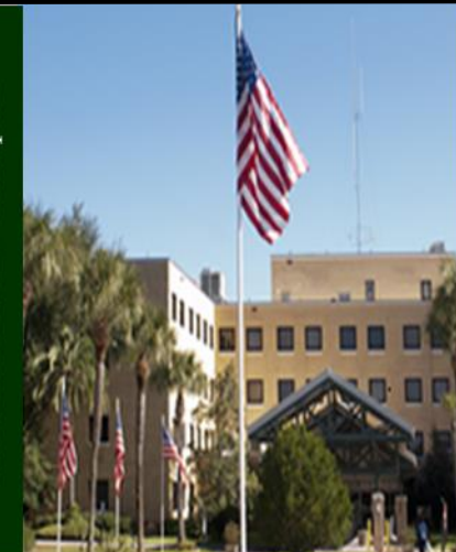
Upgrade Physical Security Malcolm Randall VA Hospital
