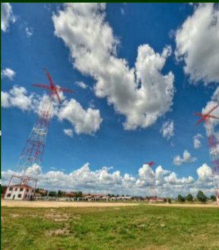
Ft. Benning Jump Towers Engineering Certification
