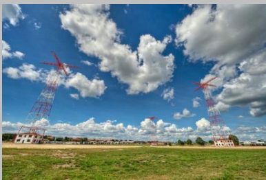
Jump Tower Inspections and Engineering Report Ft. Benning, GA
